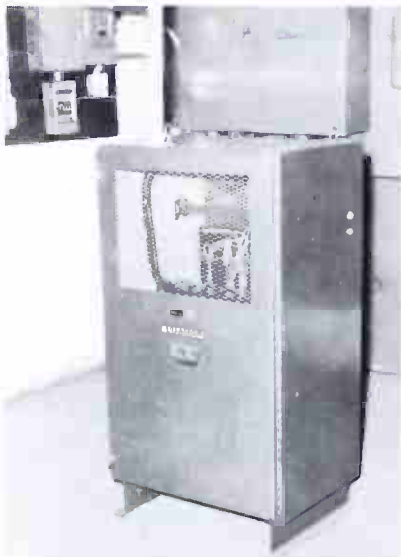
To steady the supply voltage for a mountain-top transmitter at the end of the power line, WBRE-FM installed this self-contained Solatron regulator; it keeps the output power within FCC limits.
